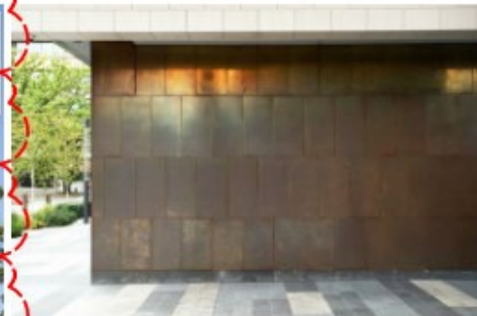
WA-MT AGED METAL SHEET CLADDING (AKOLOI, BRASS BROWN FLORENTINE CUTBACK SHEET METAL) : PLANTER BOX, ENTRY BLADE WALL & DORMER WINDOWS
